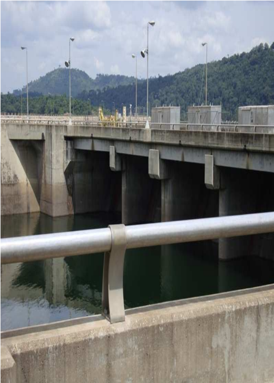
AKOSOMBO HYDROPOWER INTAKE
